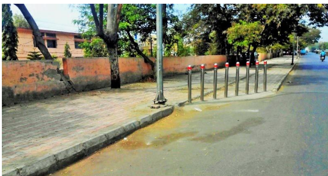
Figure 3: Ill designed cycle lane with bollards breaking the continuity
