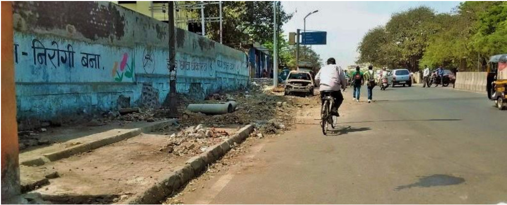
Figure 6: Cyclists and pedestrians forced to use carriage way due to lack of maintenance of cycle tracks and footpaths
